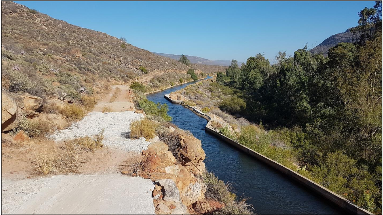
Figure 5.12: Existing Left Bank Canal looking downstream (approx. ch. 1.2 km)
