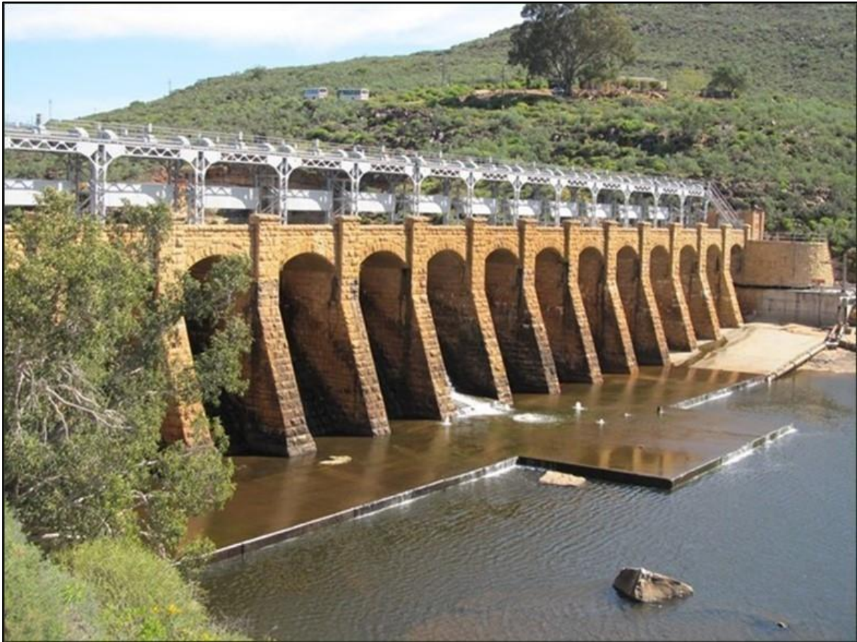
Figure 5.5: Concrete masonry Bulshoek Weir
